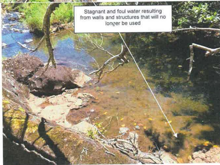
Figure 8. East Wailuanui at Koolau ditch (K-18). Stagnant water outside the west wall (top left), wall crossing stream (top right), stagnant water on the east side of the stream.
